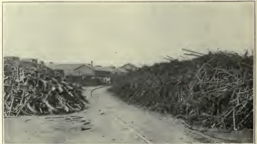
FIG. 339. MISCELLANEOUS YARDS. Scrap Yard of the Atchison, Topeka & Santa Fe Railway at Corwith.
